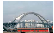
Lupo bridge, Shanghai
