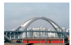
Lupo bridge, Shanghai
