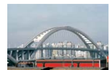
Lupo bridge, Shanghai
