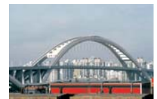
Lupo bridge, Shanghai
